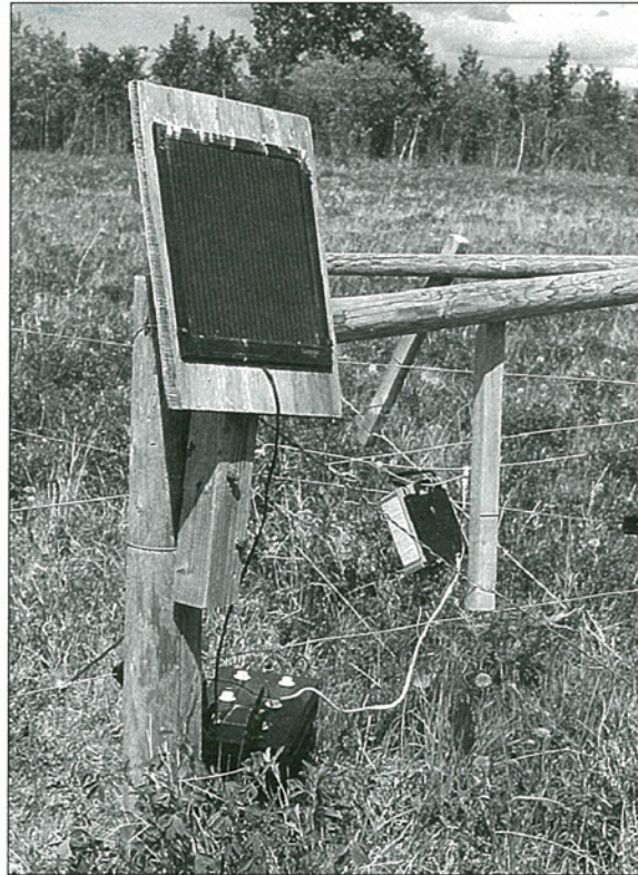
Solar-powered electric fence
